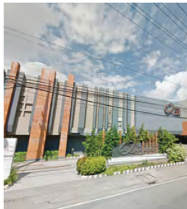
QUEUE HOTEL BINAN CITY, LAGUNA
